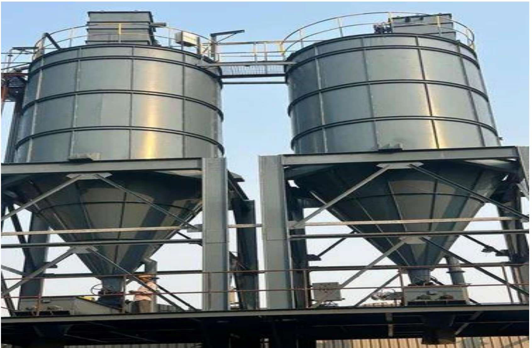
Bunker Storage Silos
